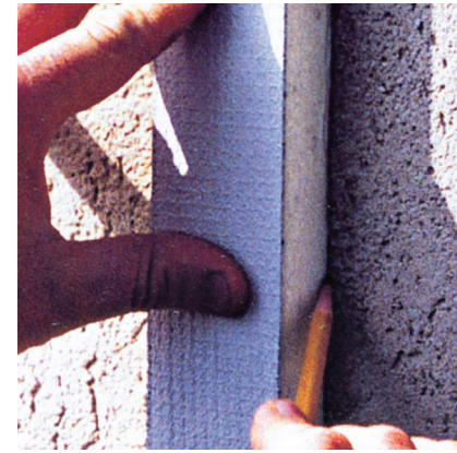
2. Use a straightedge to mark width of the required Sil-Span
