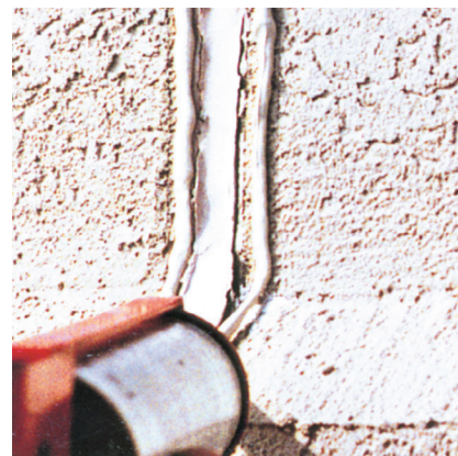
4. Apply Pecora 864NST adhesive/sealant to both sides of the joint
