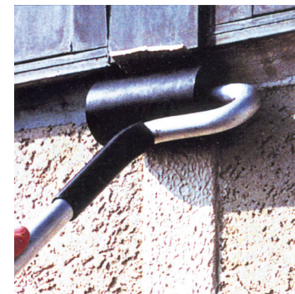
6. Remove excess caulk, trim ends, and terminate with a cap bead of 864NST
