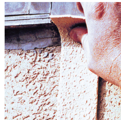
5. Apply Sil-Span to the prepared joint substrate
