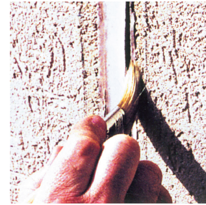
3. Clean area with alcohol and prime if necessary
