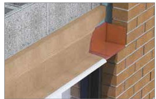
Thru-Wall shown with copper end dam (pg 42.)
